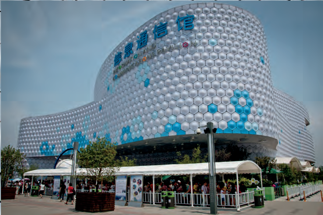
Pavilion of Information and Communications
